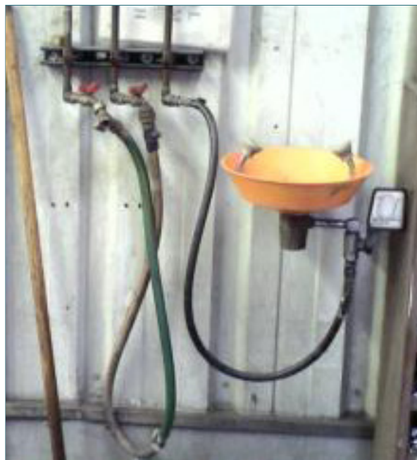
A garden hose creates a dangerous cross connection between potable and non-potable water.
